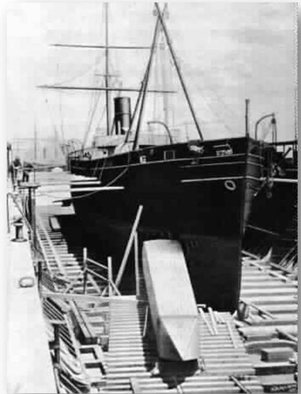
**Transfer obelisk inside the Ship cavity**
